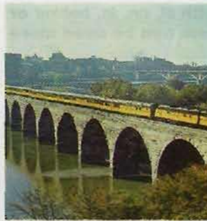
The train is going over the bridge. It's going from London to York .
